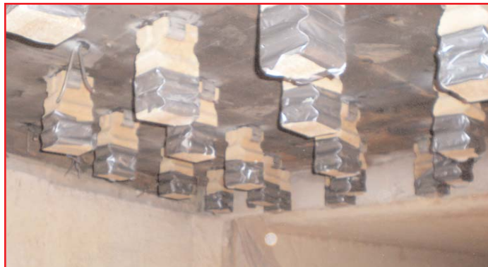
These photos show the new "top-of-the-line" ceramic hangers of the "roof" refractory repair that CORN, LP Plant Manager Andy Miller discusses in his article on page 3. The photo at left shows a close up of the metal bracket that is welded to the roof which the ceramic hanger is secured to, and the photo at right shows a series of these hangers in place.
