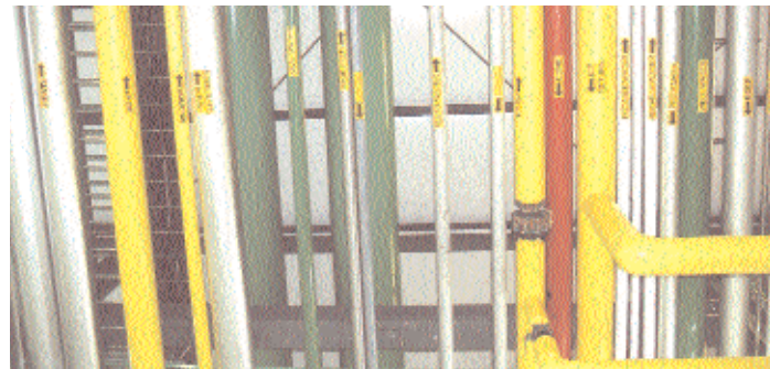
The view overhead is a maze of steam/water/product lines, all color-coded and labeled to indicate their various functions.
