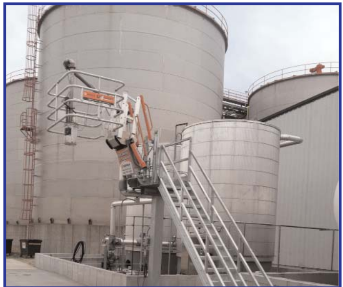
This is a picture of our oil storage, oil storage load-out, and load-out containment pad.
