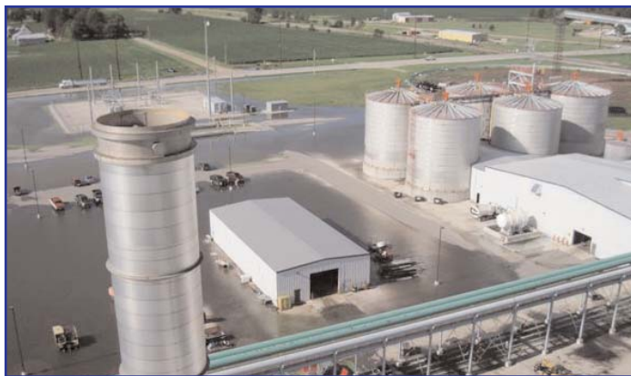
In this view looking south you can see Highway 3 and the high waters surrounding much of the CORN, LP plant on June 23rd following a 6-inch rain.
