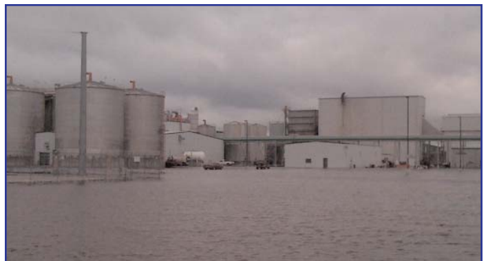
Despite having the water surrounding CORN, LP steadily getting higher with each successive rain, not a minute of production time was lost due to these unprecedented storms in June.
