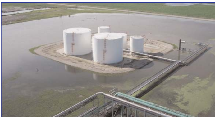
The containment berm that surrounds the Tank Farm at CORN, LP is designed to contain any leaks/spills that might occur from the tanks, but in this case the walls were holding the surrounding flood waters out.
