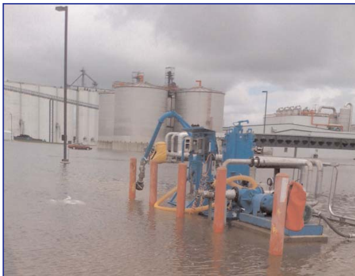
Although rising waters at one point came within 1.5 inches of the distillation containment, the CORN, LP crew was able to "Man The Pumps" in time to prevent water from entering this site.
