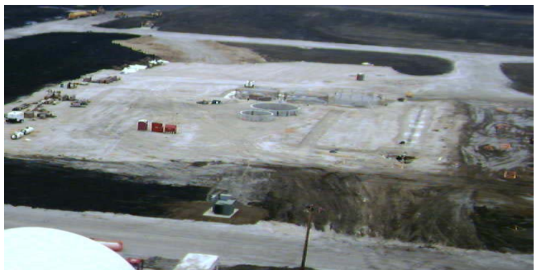
Future site of the Energy Center located on the north side of plant. Photo taken 3/25/05.
