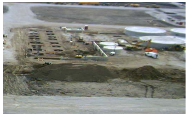
Foundation walls are erected for the processing building. Photo taken 4/05/05.
